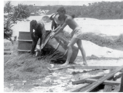
Mixing concrete for foundations January 1950. L-R Billy Ball, Morgan Evans, Col Willett
